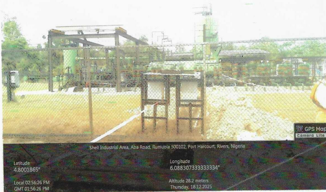
View of spill area in front of the Flow Station
